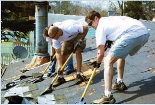
The existing roof coverings, whether they're shingle, slate or tile and rolled material, should be removed down to the existing plywood or sheeted roof deck. Per shingle manufacturer specifications, if shingles are installed over any of these roofing materials the warranty will become null and void. Always follow the manufacturer's product specifications for roof replacement.
