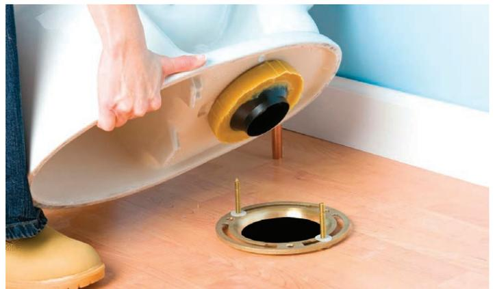
Next, start assembling your new toilet. First, install a new wax ring onto the waste horn, which is the part protruding from the bottom of the toilet that connects to the flange. If you had stored your wax ring in a cool place, allow it to warm up a little bit before installing it to make it easier to work with. Remove the rags to unplug the drain hole, and gently place the toilet over it, aligning the wax ring
