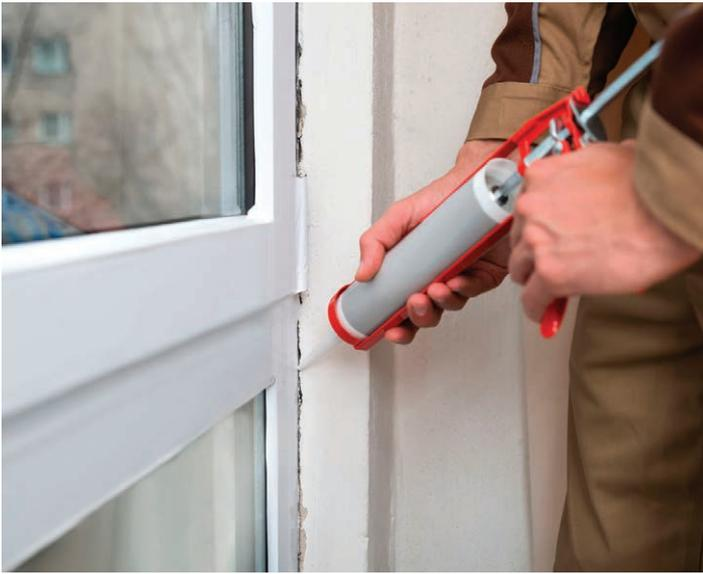
If the old caulk is damaged or deficient, remove it with a scraper or sturdy putty knife. In these areas and in areas that are totally devoid of caulk, clean the adjacent surfaces, sand them smooth, and spot-prime if any bare wood shows. This will help your caulk adhere properly to create a weather-tight seal.
